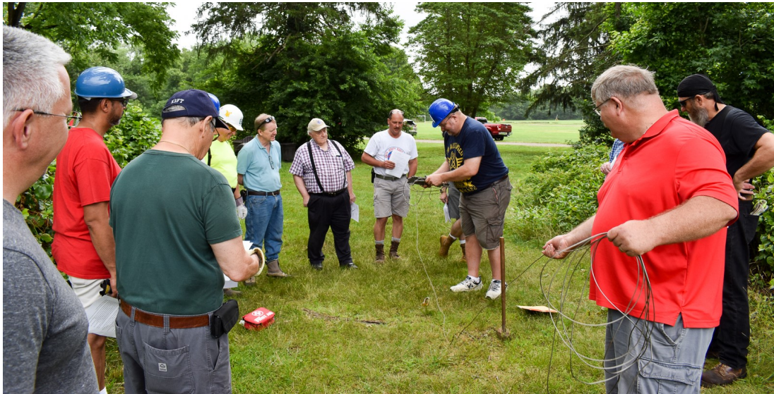
Ken, K2WB going over guying and tower installation.
