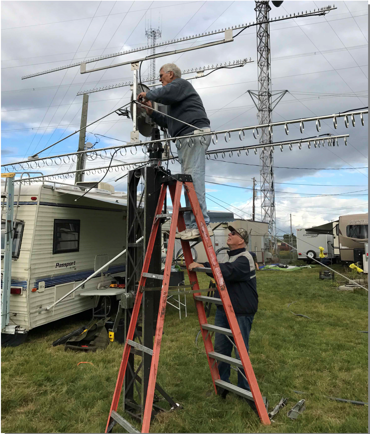
Ray, N3RG and Bob, W2SJ, putting the final touches to the Microwave stack before raising the tower on High Knob, Hawley, PA just before the 2017 ARRL VHF/UHF QSO Party (contest).
