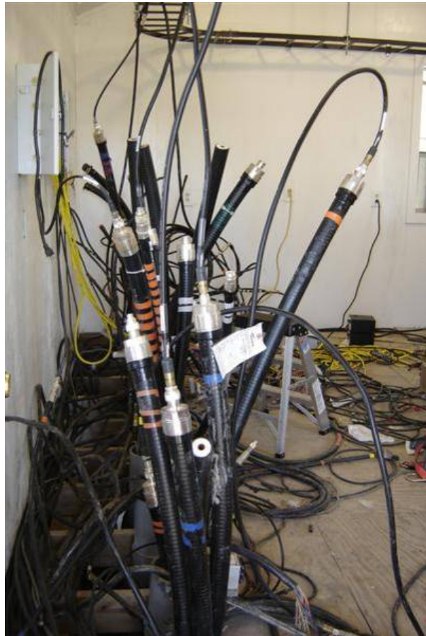
Underground run to switch shack
