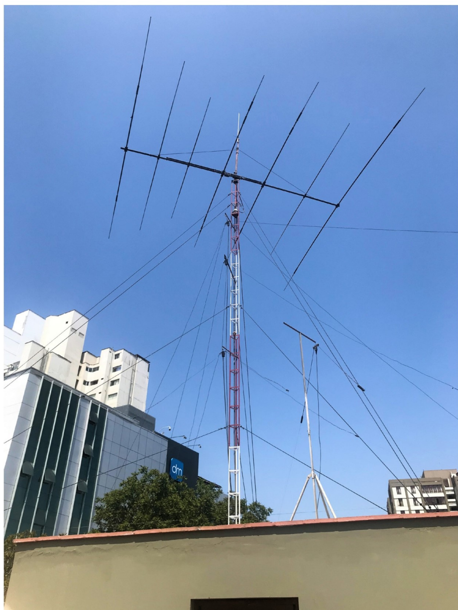
Father Ed's rooftop antenna farm with a Hy-Gain TH-7 tribander and multiple inverted V antennas. [Courtesy of Ed Schmidt, OA4SS]
