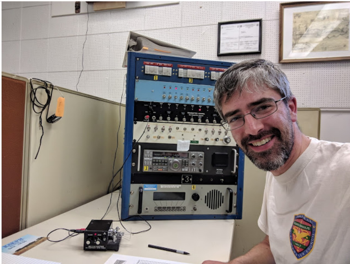
Jeff Kabel/AA6XA at Position Three. Photo Courtesy of Jeff Kabel.
