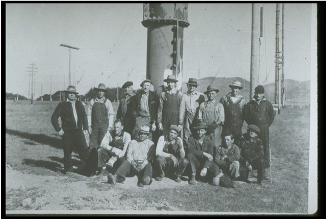
The BOLINAS RADIO riggers from back in the day. They are standing at the base of one of the 300 foot Marconi steel towers. These hardy souls climbed these towers in every hour of the day, and in every kind of weather, to maintain and repair the antenna system at Bolinas. We sure could use their help today!
