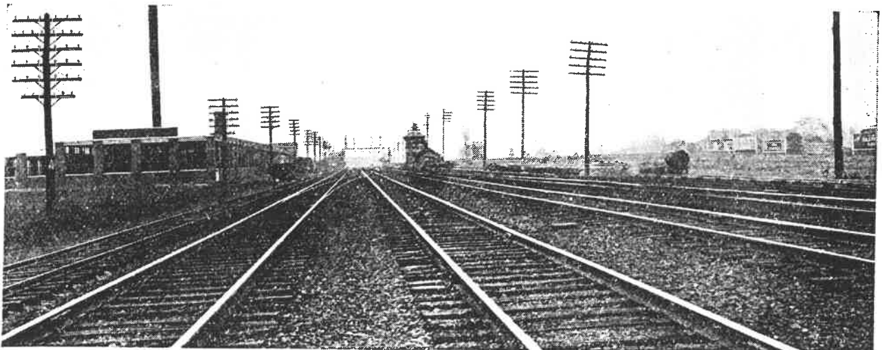
A stretch of standard four-track roadbed on the New York division showing the double line of poles carrying railroad telegraph and telephone wires. The Railroad believes in the old adage, "Do not put all your eggs in one basket." In the event of storm or emergency, immediate connections may be made between wires on these two lines, providing a reserve wire service sufficient to meet practically every demand made upon it.
