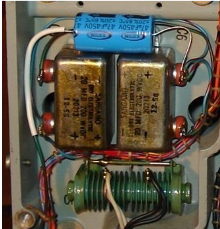
New 47uF Capacitor Replaces C5 and C6
