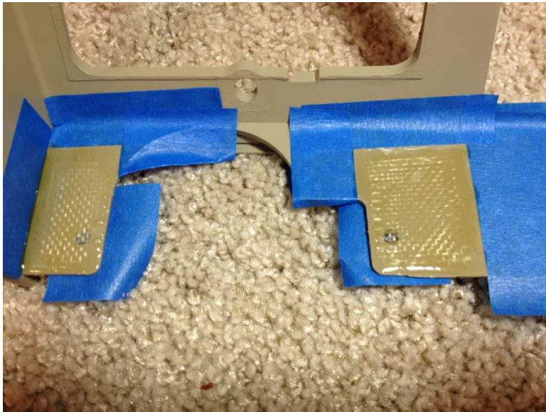
Resin applied over fiberglass patch.
