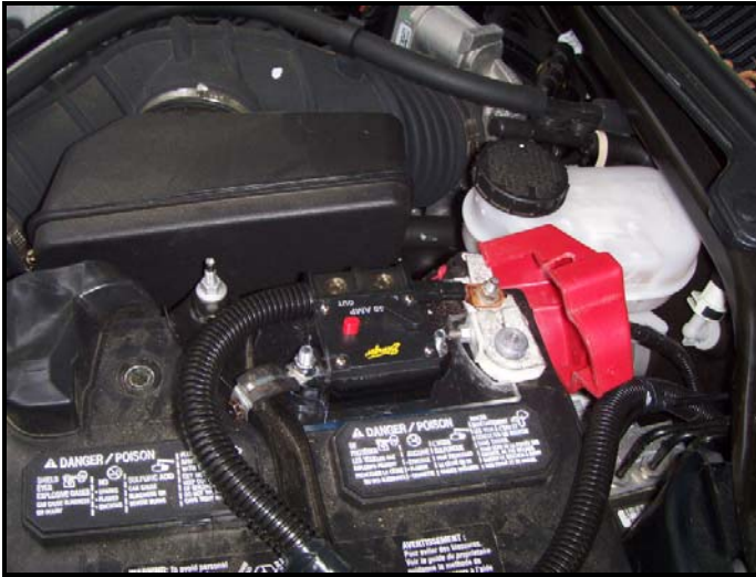
50 Amp breaker bolted to Plexiglas and that is glued and bolted on top of battery, #6 wire run to breaker panel through firewall and under carpet
