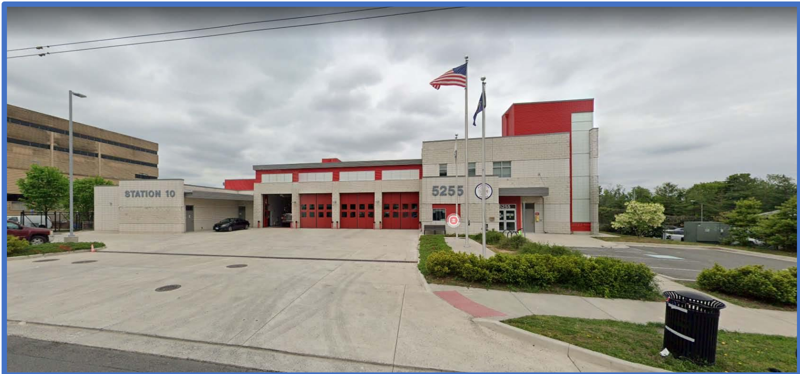
Alexandria Fire Station 210, 5255 Eisenhower Avenue
