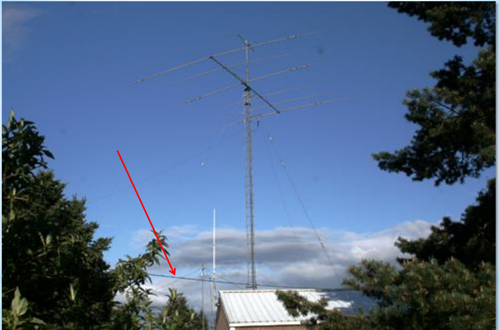
Power line noise at W7VO
