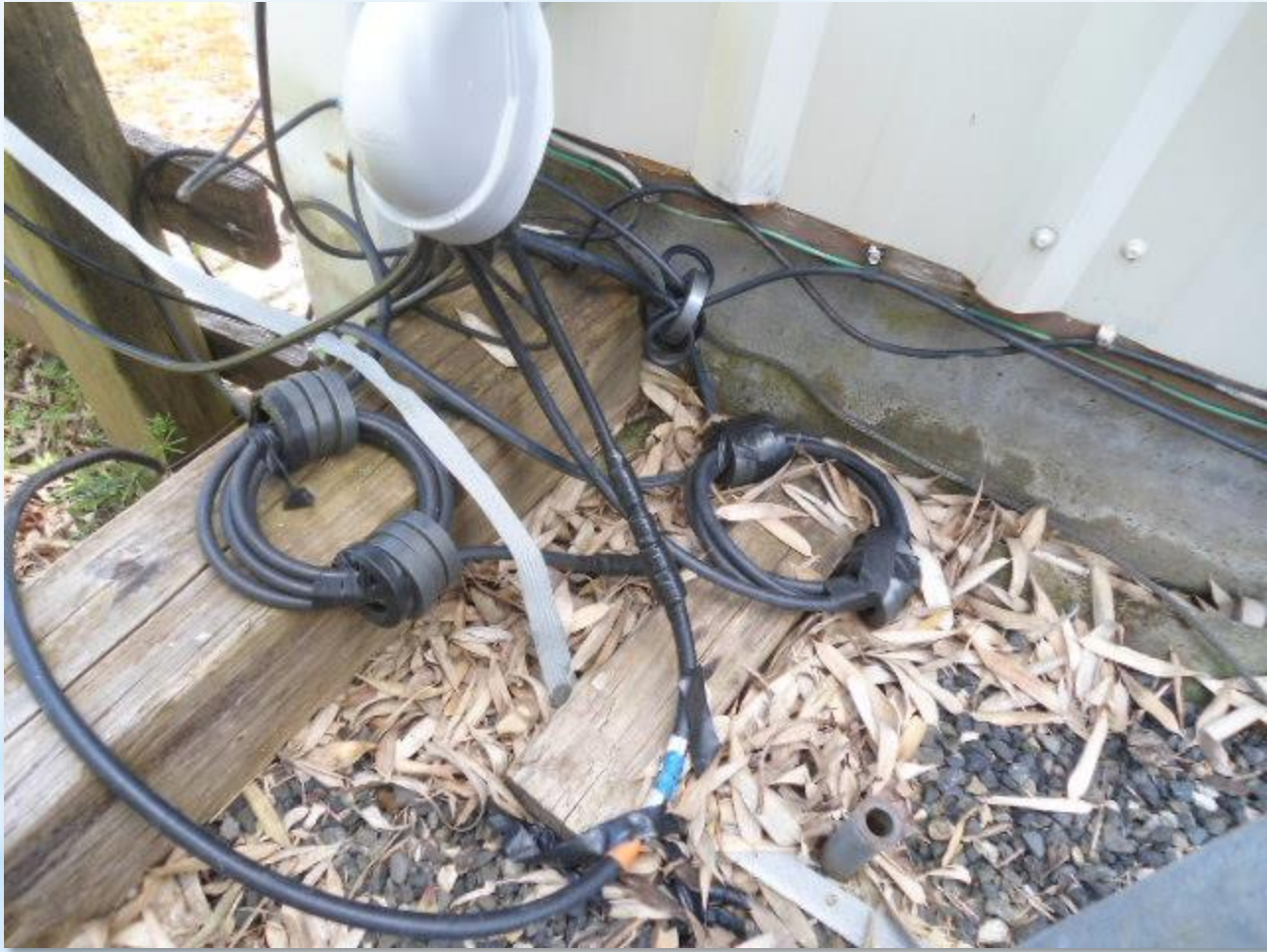
Common Mode Chokes on lowband antenna feedlines at W7VO
