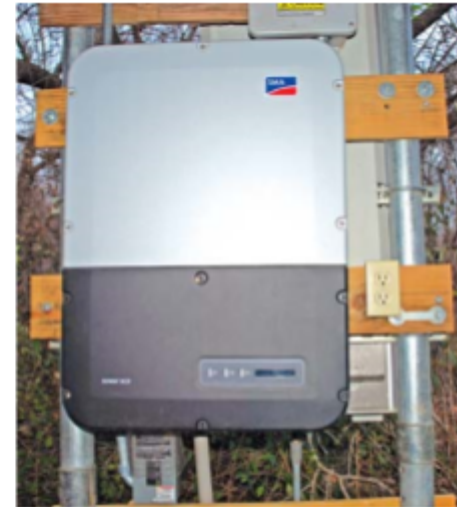
Figure 1 — A grid-tie string inverter with a grid-down secure power outlet on the right.
