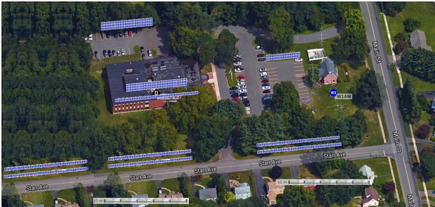
This 576 panel array of 277W panels yields 160 kW and should equal an annual 190 MWhr total consumption
