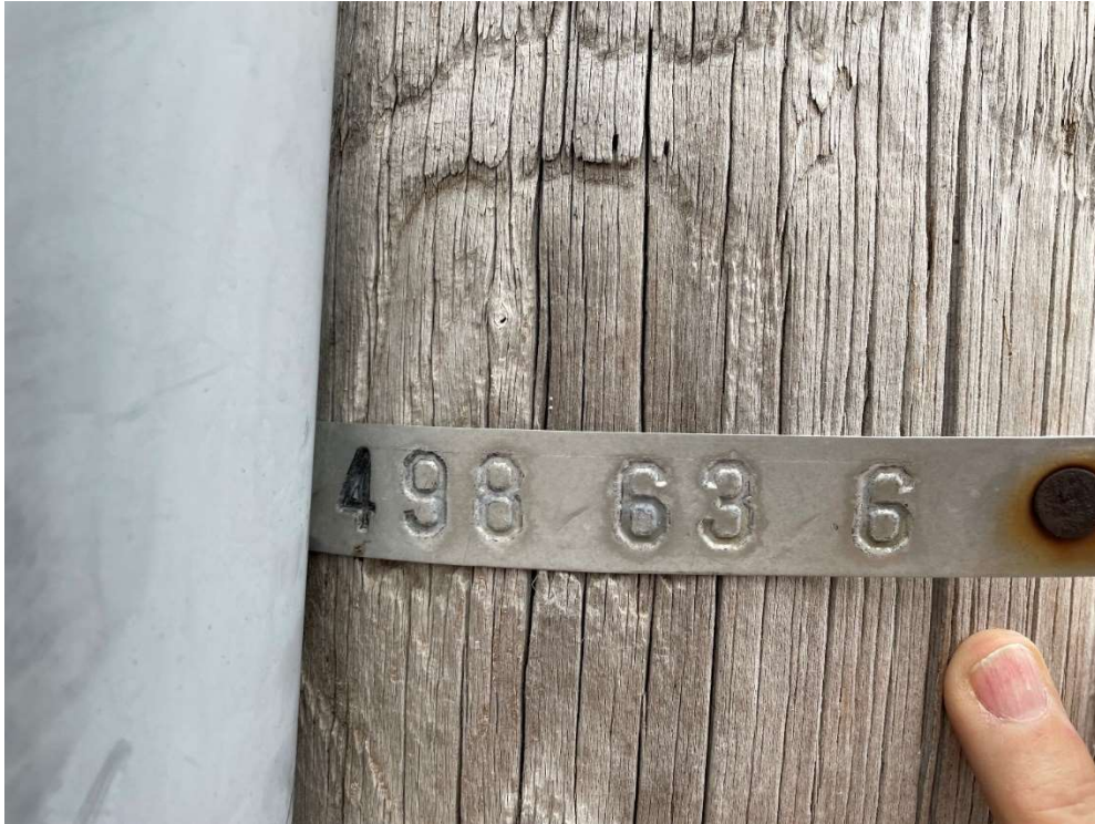
Figure 3 – Source of Interference: Pole 498 63 6 at 2924 Highway 157
