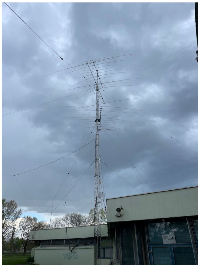
<- Antennas at the 9A1A Headquarters Station
